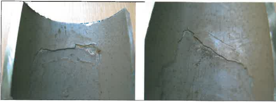
Figure 4. Boiler waterwall tube – flaky deposits on the internal surface
